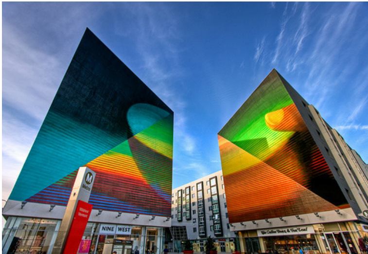
Figure 15- Transit-oriented development above Wilshire/Vermont Metro Station
