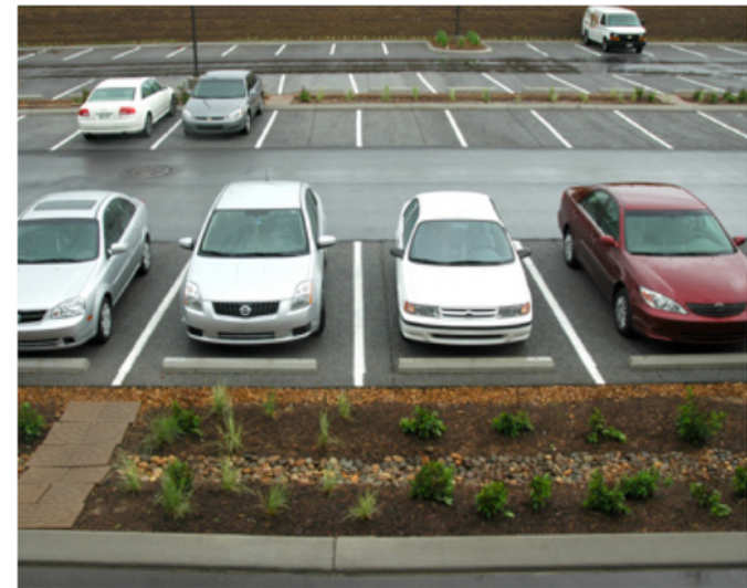
Bioswales and Vegetation (Left - Figure 25), Permeable Pavement in Parking Lane (Top - Figure 26), and Permeable Pavement and Bioswales in Surface Parking Lot (Bottom Right - Figure 27)
