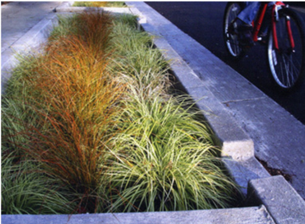
Figure 17 - Sidewalk Swale for the Bio Street. Source: Media Project Online, available at http://mediaprojectonline.org/heavyweather/heavyweather-images/swale002.jpg
